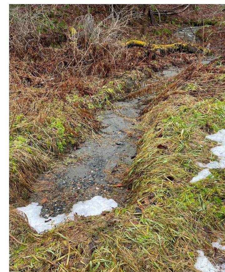
Culvert Outlet at Stream Photograph
